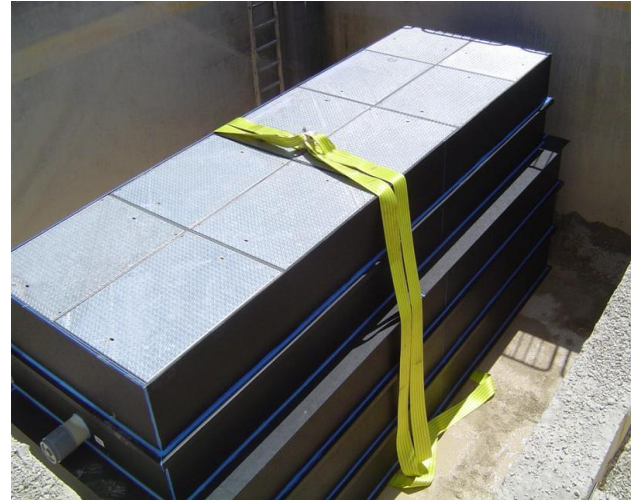
Installation of the plant in the test pit
