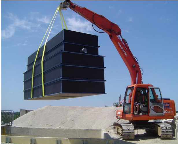
Handling of the plant in the test pit
